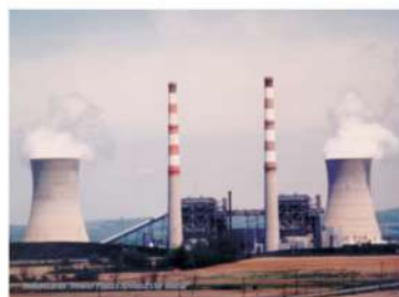
▲ Figure 1.1 Steam Power Plant
