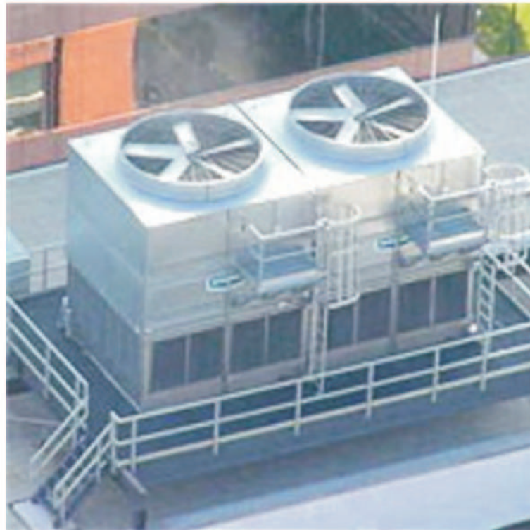
▲ Figure 6.3 Parts of an Induced Cooling Tower
