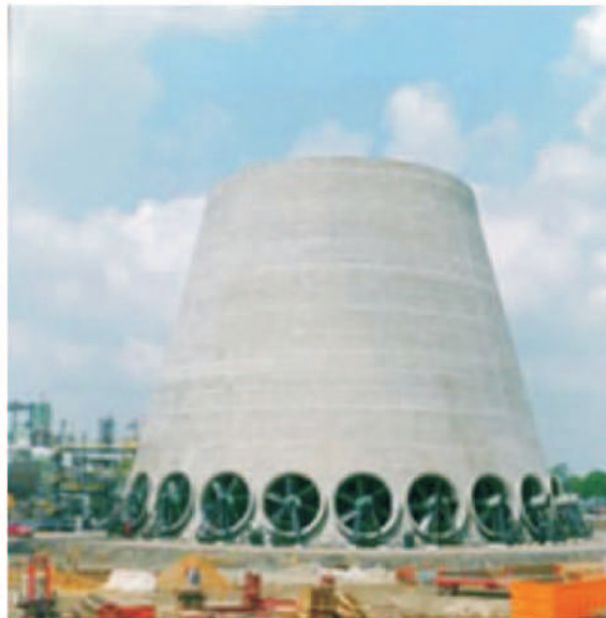
▲ Figure 6.7 Forced Cooling Tower
